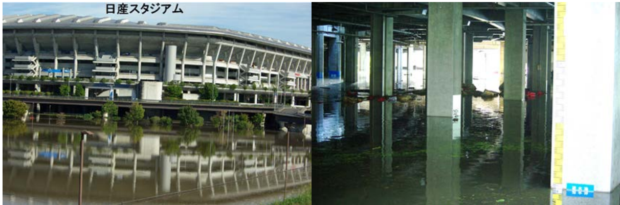
Photo 2: Flooding around International Stadium Yokohama (left) and stored flooded water under the stadium (right)
